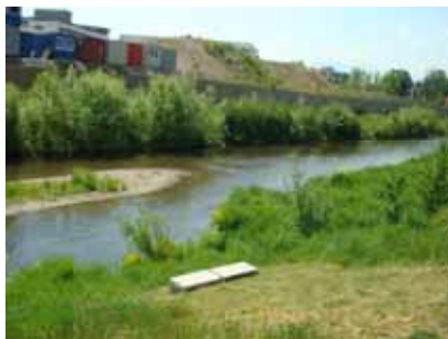
Extension of hospital related to river renaturation...
